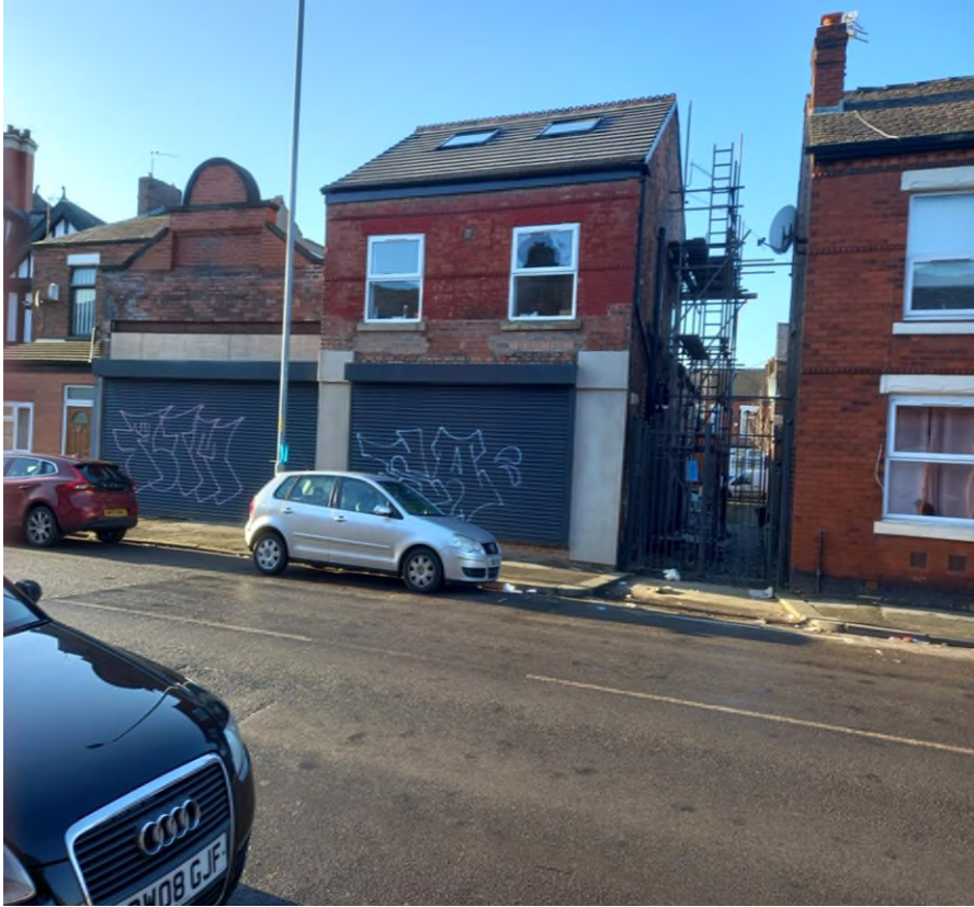
Existing site – front view
