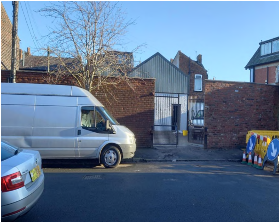
Existing site – rear view
